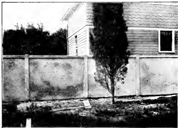
Fig. 140—Cement Mortar Fence Complete
